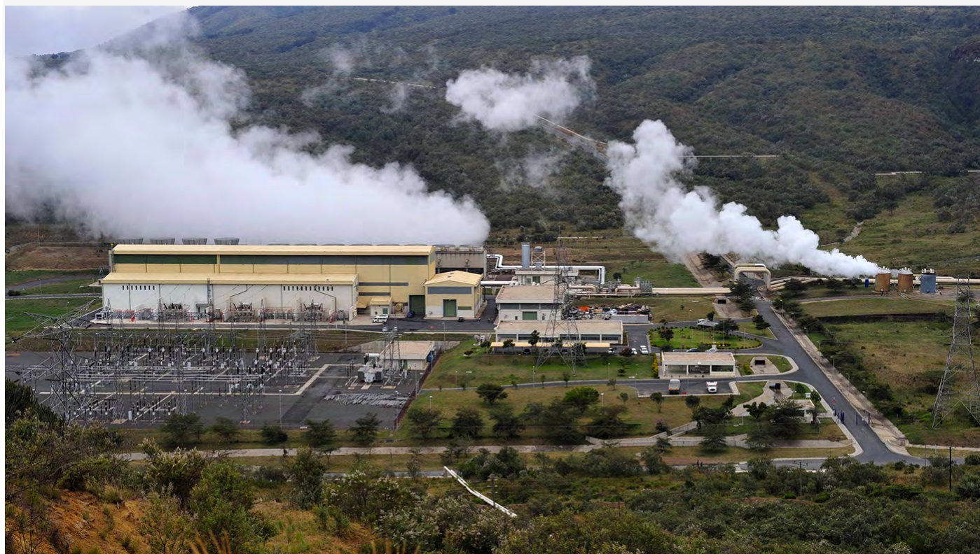
Olkaria Geothermal Power Station.
