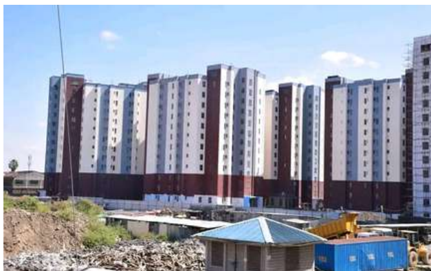
Mukuru Met Site Social Housing Project in South B, Nairobi
